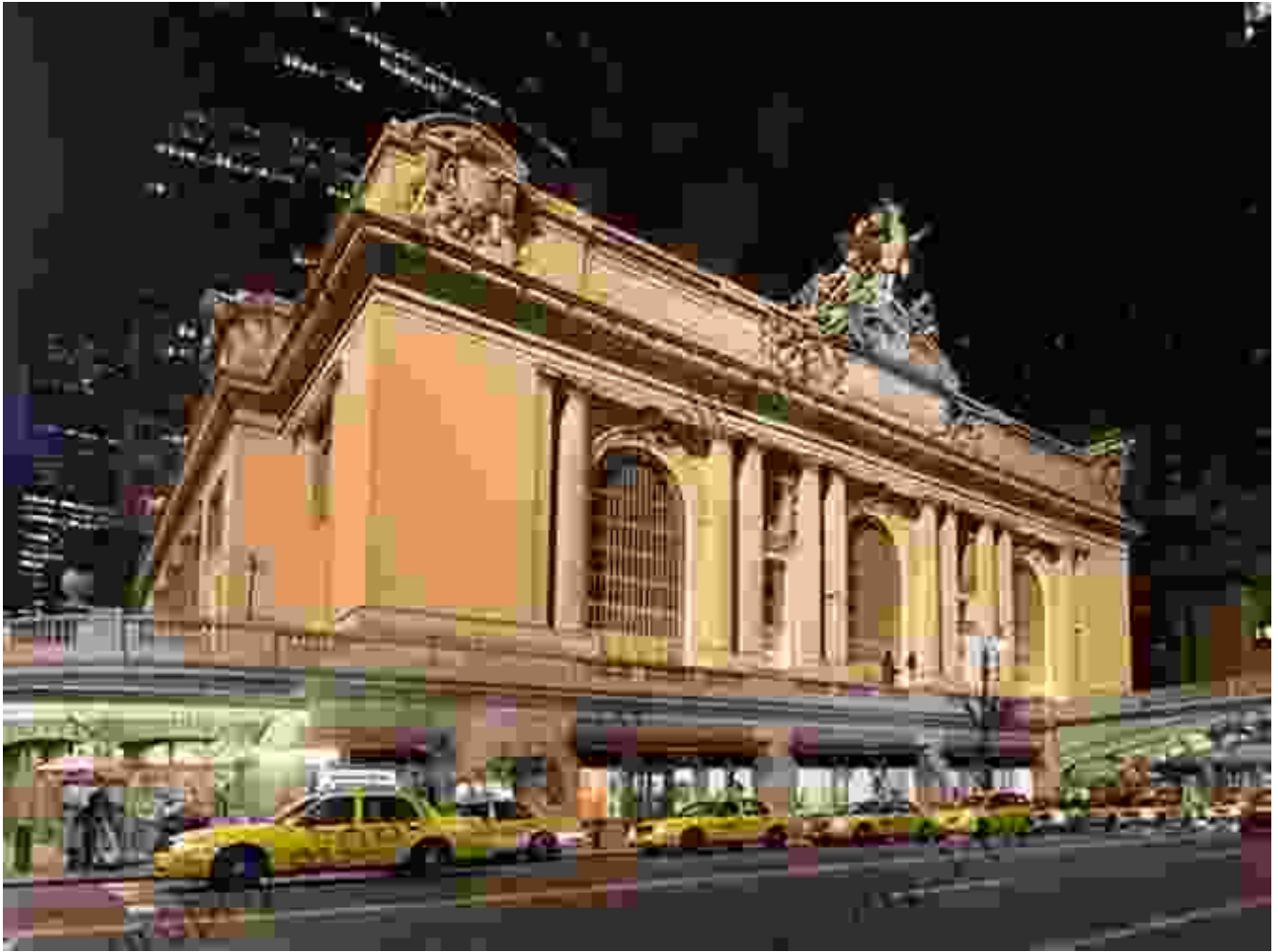
Grand Central Terminal
